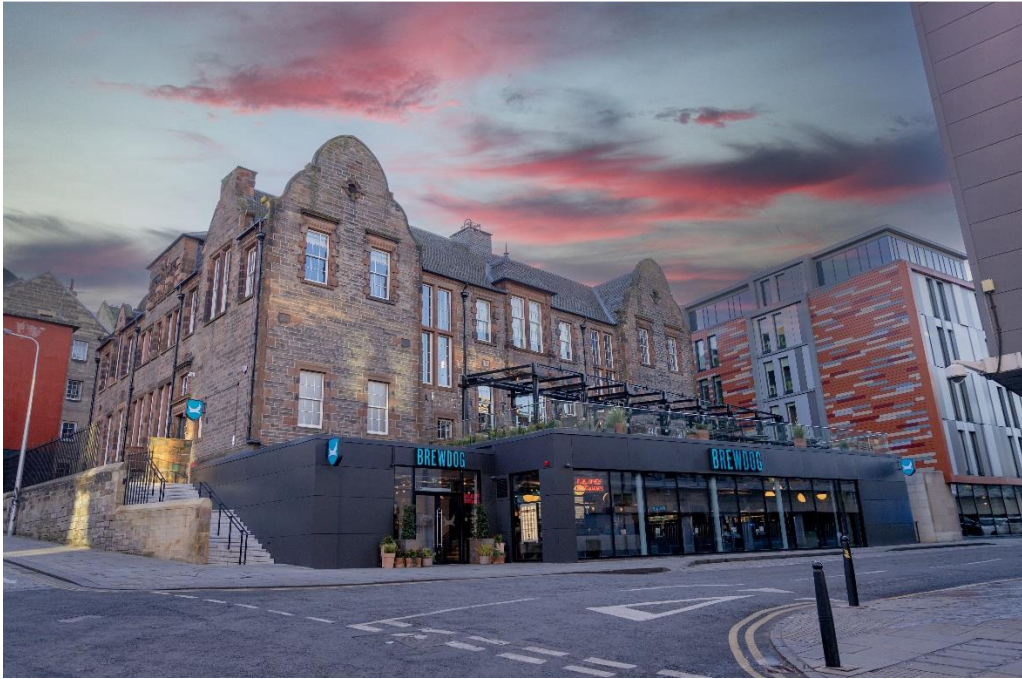
Image 7: Existing Canopy occupying the full width of the terrace
